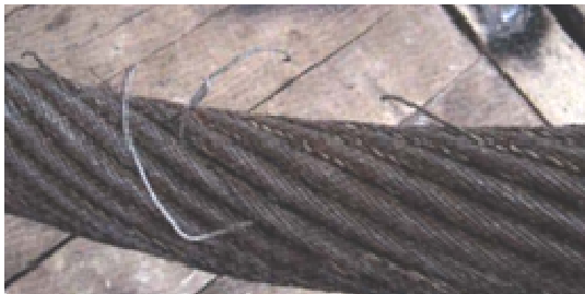
g. Internal Broken Wires in the Outer Strands of a Multi-Strand Rope
