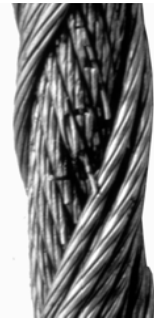
d. Broken Wires in Second Layer of Strands
