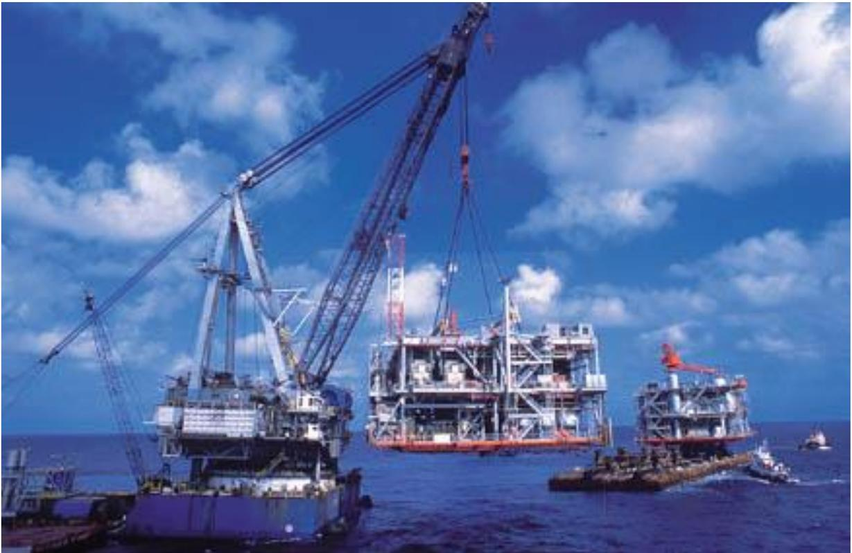
Figure 1. The Heavy Lift Vessel DB-50 is shown here lifting the North module of the Petronius compliant tower into place. The [ill fated South module](#) is visible in the background.
