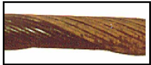
Figure 7 Corrosion in the second and third layer of the rope
